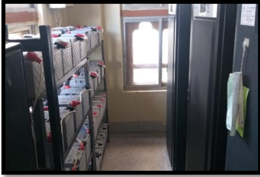
(40KVA UPS with battery)
